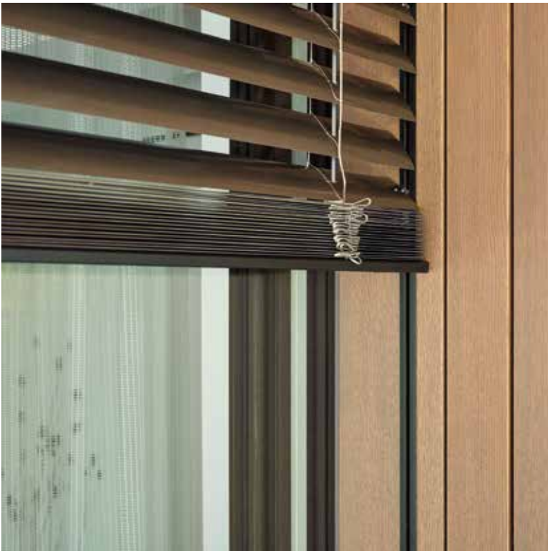
Venetian blind with concealed guide rail embedded/plastered in the wooden panelling.
